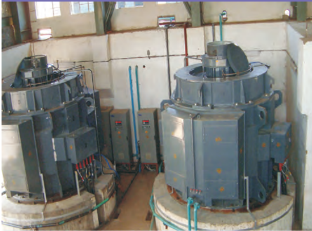
12.8 MW Synchronous Motors
