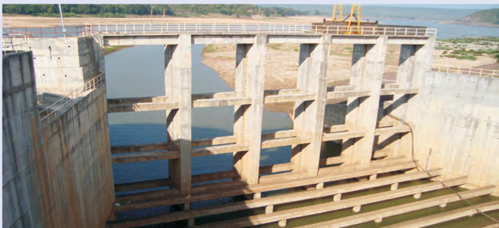
Forebay Structure at Intake Pumping Station
